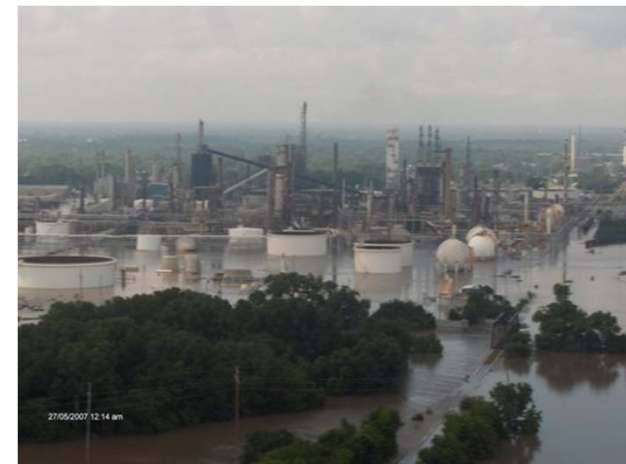
Coffeyville Refinery Kansas July 2007
