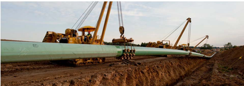
Enbridge Pipeline Replacement Project $1.6 billion in Indiana and Michigan
